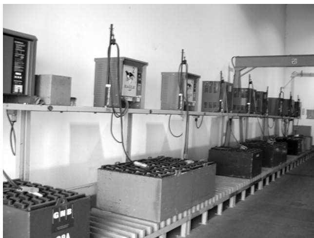
Batteries and battery chargers for electric forklifts.
