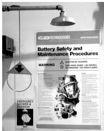
Example of a battery safety sign and emergency body shower in a battery charging room.
