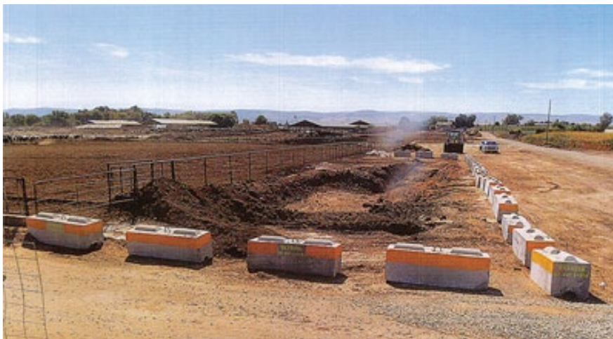
The edges around manure storage sites can appear deceptively solid. Here is one possible solution that can prevent entry. Photo: L&I.
