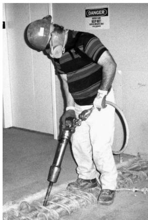
**FIGURE 2. Hand Demolition:** Handheld concrete demolition involved the use of a small jackhammer or reciprocating gun with interchangeable chipping or rivet busting head to remove excess concrete from overpours, splashovers or when concrete forms did not meet.
