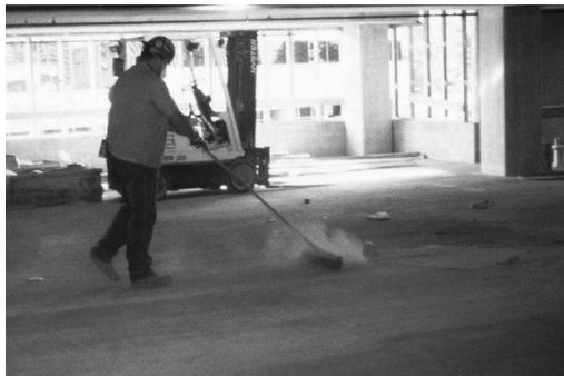
**FIGURE 1. Cleanup:** Cleanup involved the removal of construction debris, particularly settled dust, using brooms, shovels, and occasionally a backpack blower. There was often frequent interruption of the cleanup task to move obstructions out of the way.
