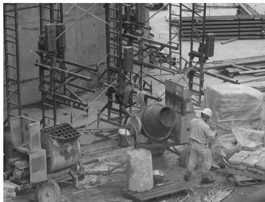
**FIGURE 4. Concrete Mixing:** Concrete, mortar, and grout are mixed, usually by the hod carrier on a brick mason crew. Typically mortar was mixed 3-4 times in a shift, with each session taking about 10 minutes. On two occasions, grout could not be delivered to the site and it was hand mixed, resulting in a fairly continuous period of mixing.
