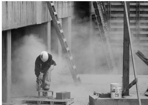
**FIGURE 3. Concrete Cutting:** Concrete block was cut using a handheld gasoline or a table-mounted masonry saw. The handheld saw was always used outside, and cutting was intermittent and always dry, whereas the table-mounted saw was used both inside and outside on scaffolding, usually cutting with at least some water spray to the blade and sometimes continuously for several hours.
