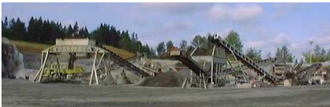
Figure 1: Portable screening and crusher operation
