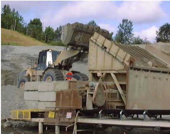
Figure 2: Loader feeding shaker
